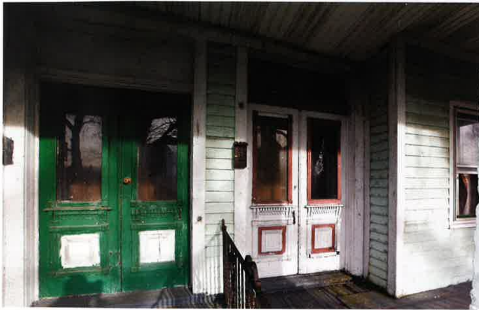
Details of the vacant structure; archival images of Joanne and Gloria Riforgiato
